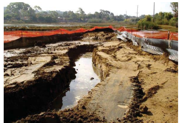
Shaping the channel
